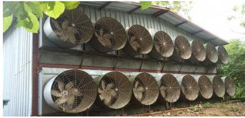
Gambar 12. Exhaust Fan (Blower)
